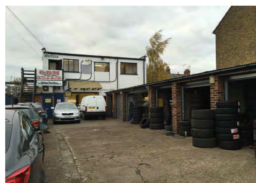
IMAGE OF 7/9 LANSDOWNE AVE (APPLICATION SITE)
